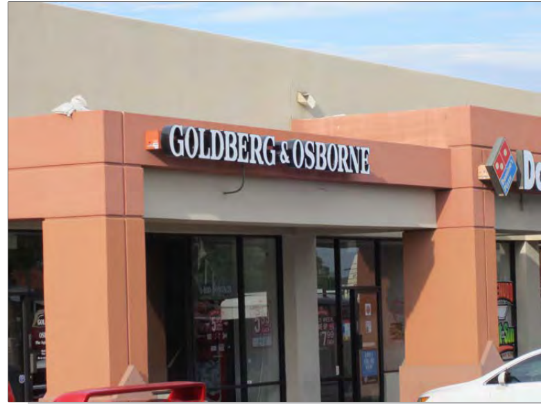
Typical Pan Channel Lettering and Logo Internal Illumination Mounted on Raceway to Building
