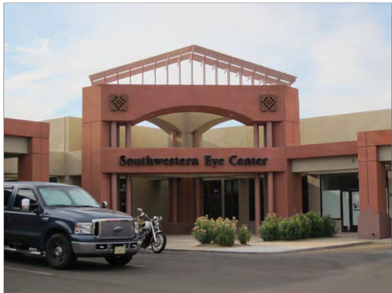
Typical Reverse Pan Channel Lettering and Logo Backlit "Halo" Illumination Peg Mounted to Building
