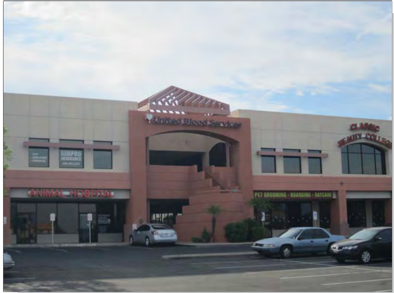
Typical Pan Channel Lettering and Logo Internal Illumination Mounted on Raceway to Building Two Story Tenant Space
