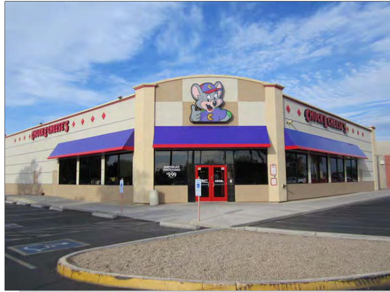
Typical Pan Channel Lettering and Logo Internal Illumination Flush Mounted to Building
