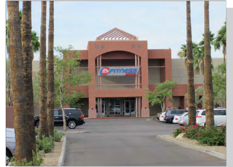
Typical Pan Channel Lettering and Logo Internal Illumination Mounted onto Specialty Metal Background to Building
