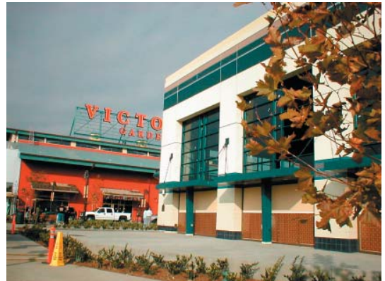
Unique glazing is used to enhance the theme of the building
