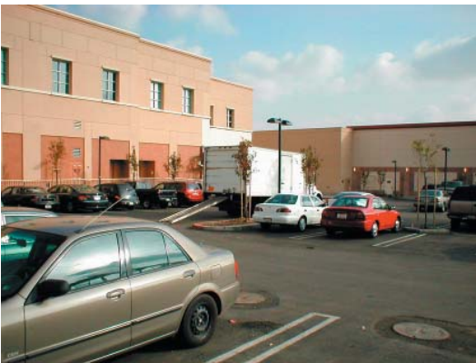
360 ° architecture used within a loading court
