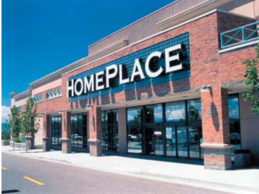
Ceramic tile utilized at building entrance.
