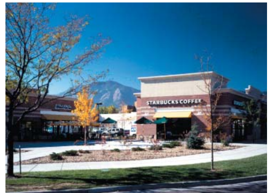
Unique Pad building architecture utilized by national Tenants.
