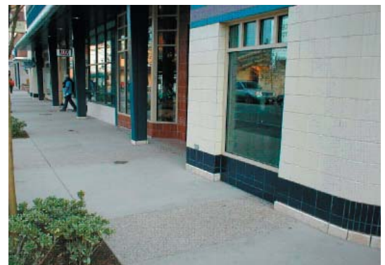
Ceramic tile provides a colorful base material for the building facade.
