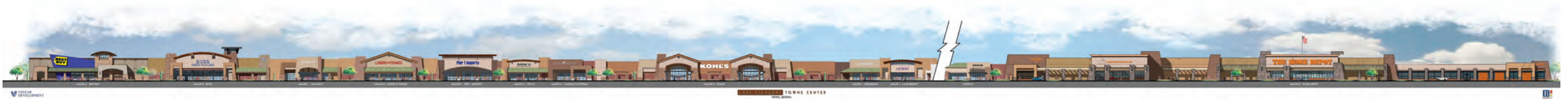
BUILDING ELEVATION CHARACTER
